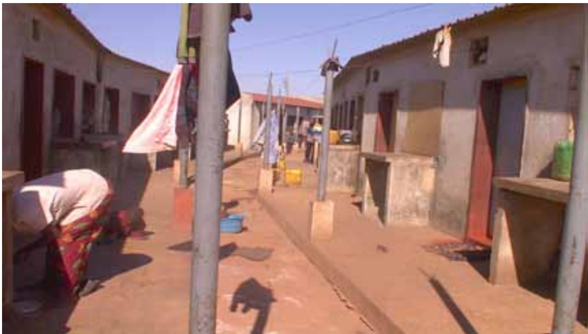
Another view of the market structure serving as officers' accommodation
